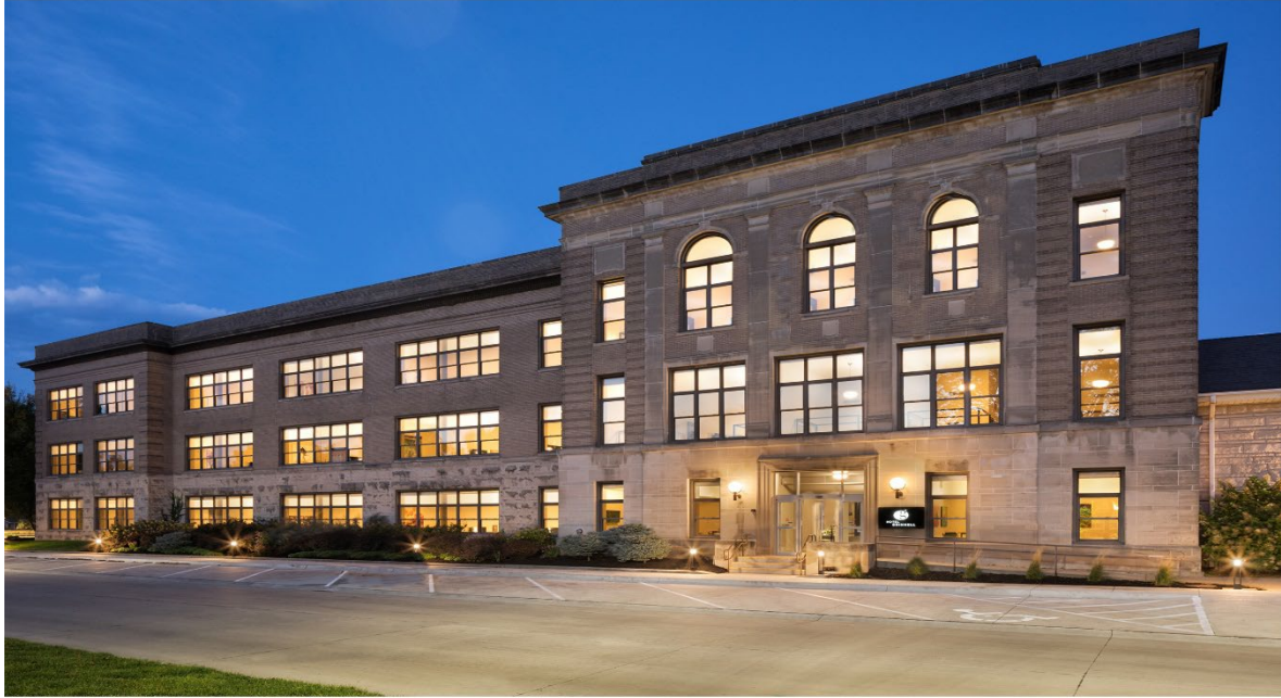
Photo of Hotel Grinnell East Façade in evening. This photo shows the conversion of the former Grinnell Junior High School into a boutique hotel-events center. 9/11/17
