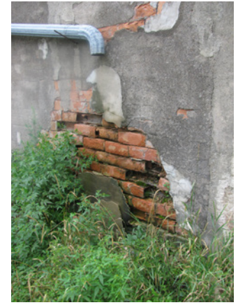
Deferred roof maintenance and improper downspouts can cause significant issues due to water infiltration.
