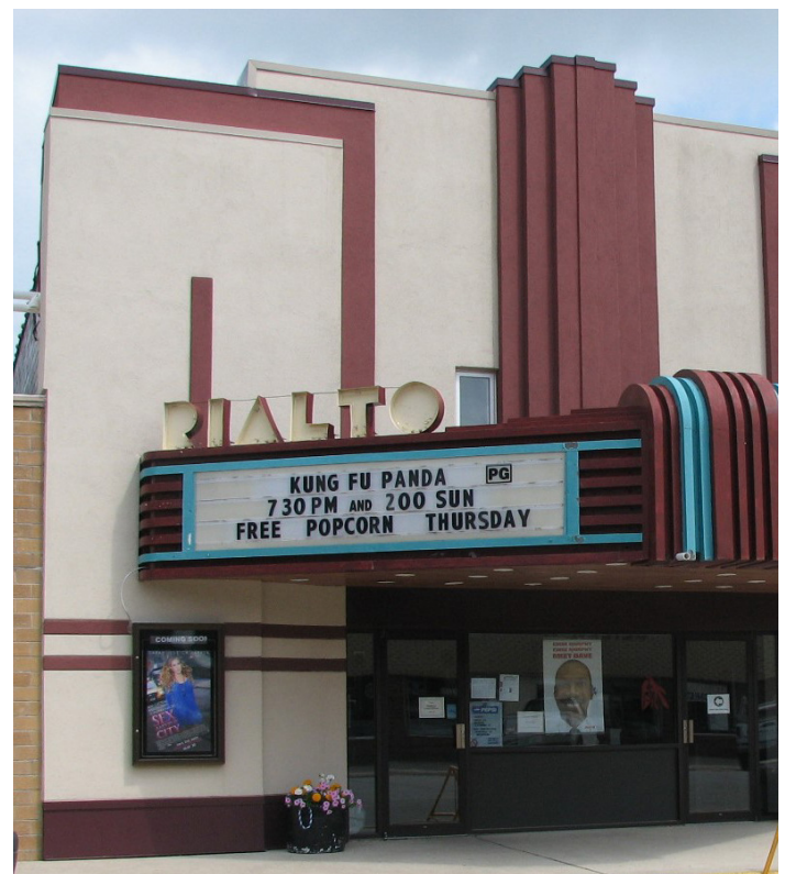
Widespread use of stucco contributes to the distinctive streamlined character of this theater.
