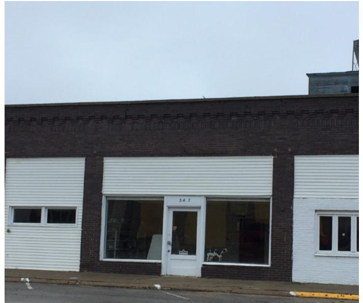
Vinyl siding creates a residential appearance and should not be used as infill or primary material on downtown buildings.
