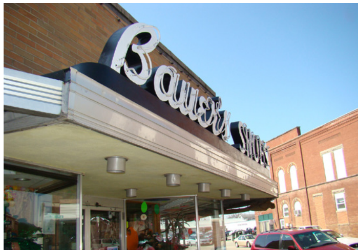
This integrated canopy signage is a character-defining feature of this mid-century building.
