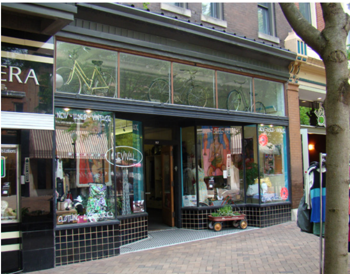
This intact historic storefront features a stepped recessed entry, bulkhead tile, and thin metal window frames.
