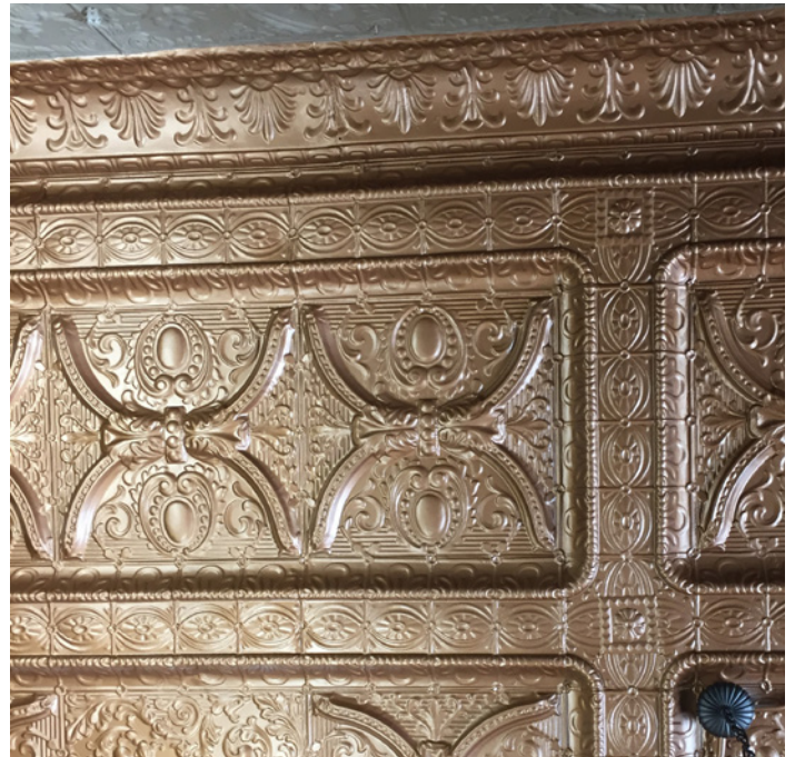
Restoration of historic tin ceilings can create a unique focal point for interior spaces.
