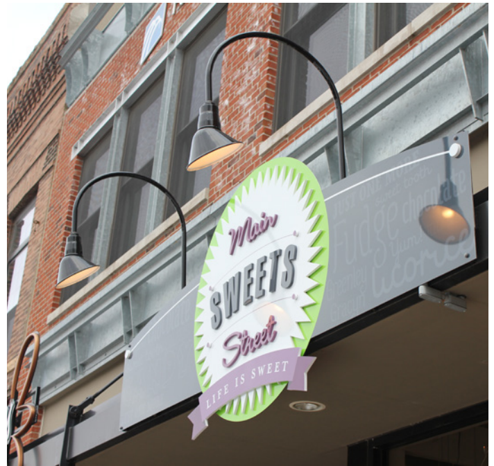
Gooseneck lighting is a great way to provide signage illumination and increase curb appeal.
