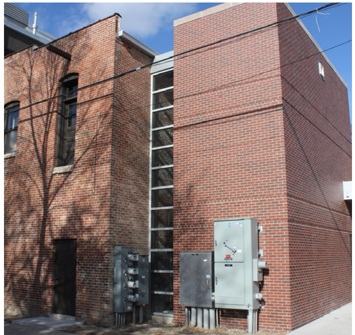
A glass hyphen joins this rear elevator addition to the original building, and distinguishes it from the historic construction.
