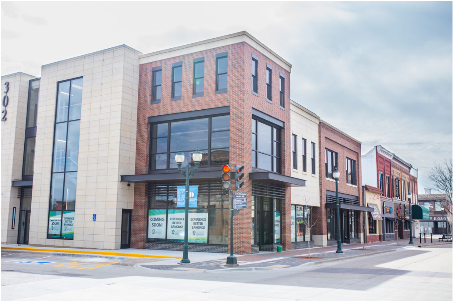
This example of compatible new construction divides the facade into multiple storefronts, maintains proportions similar to other downtown buildings, and utilizes quality, traditional materials.
