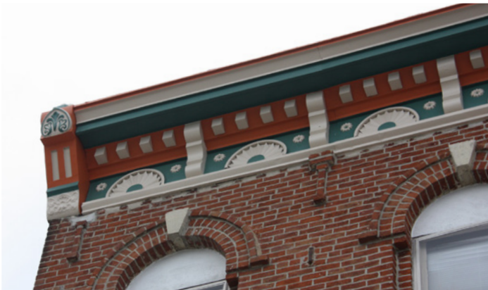
Wood cornices are often painted to highlight elaborate details.
